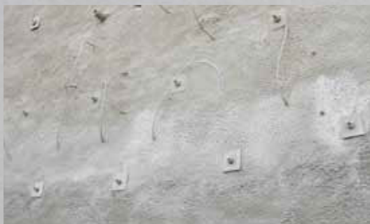
Nailed shotcrete wall
