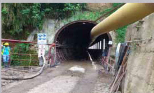
Shotcrete for tunneling/mining
